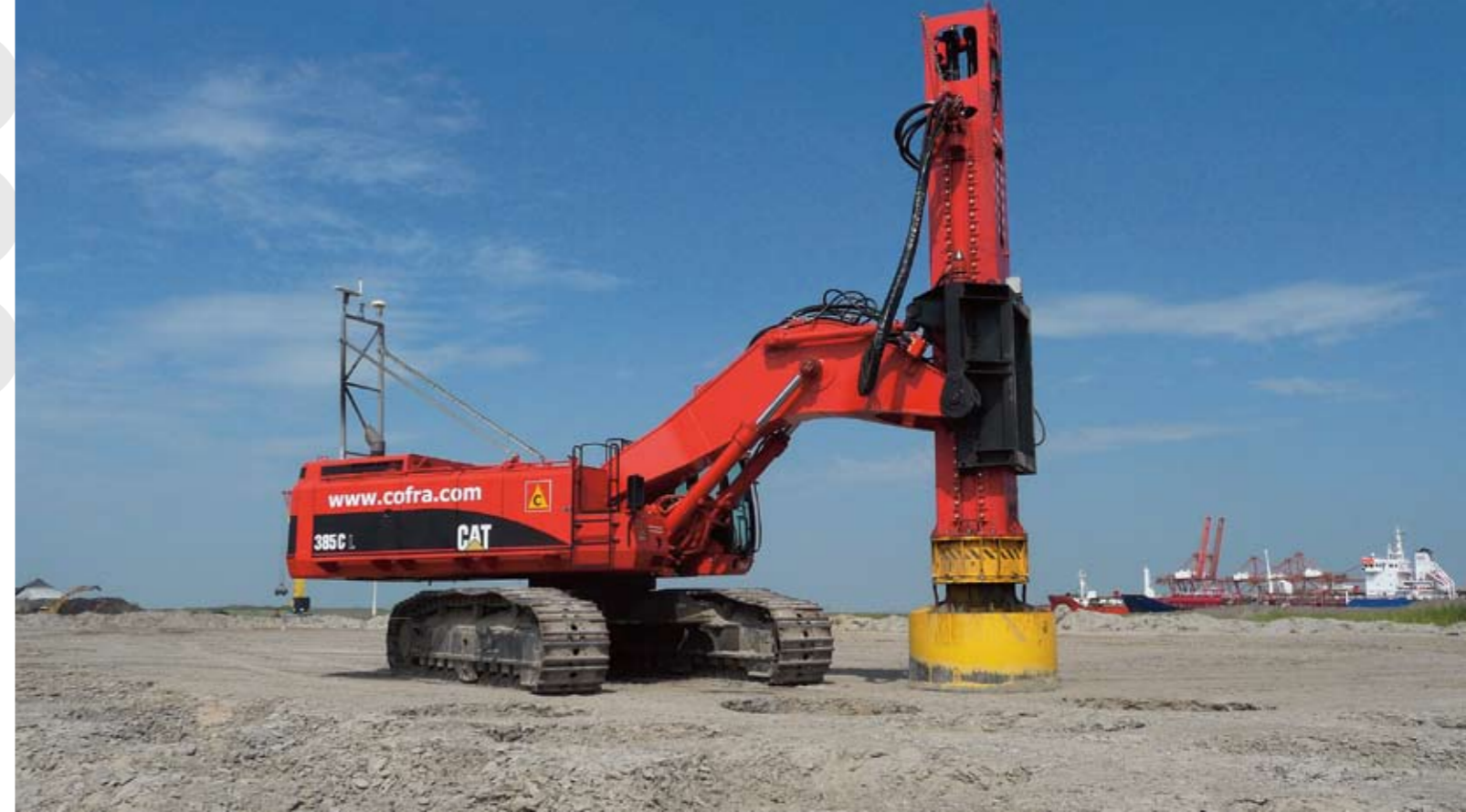
Compaction at the Vopak terminal site
