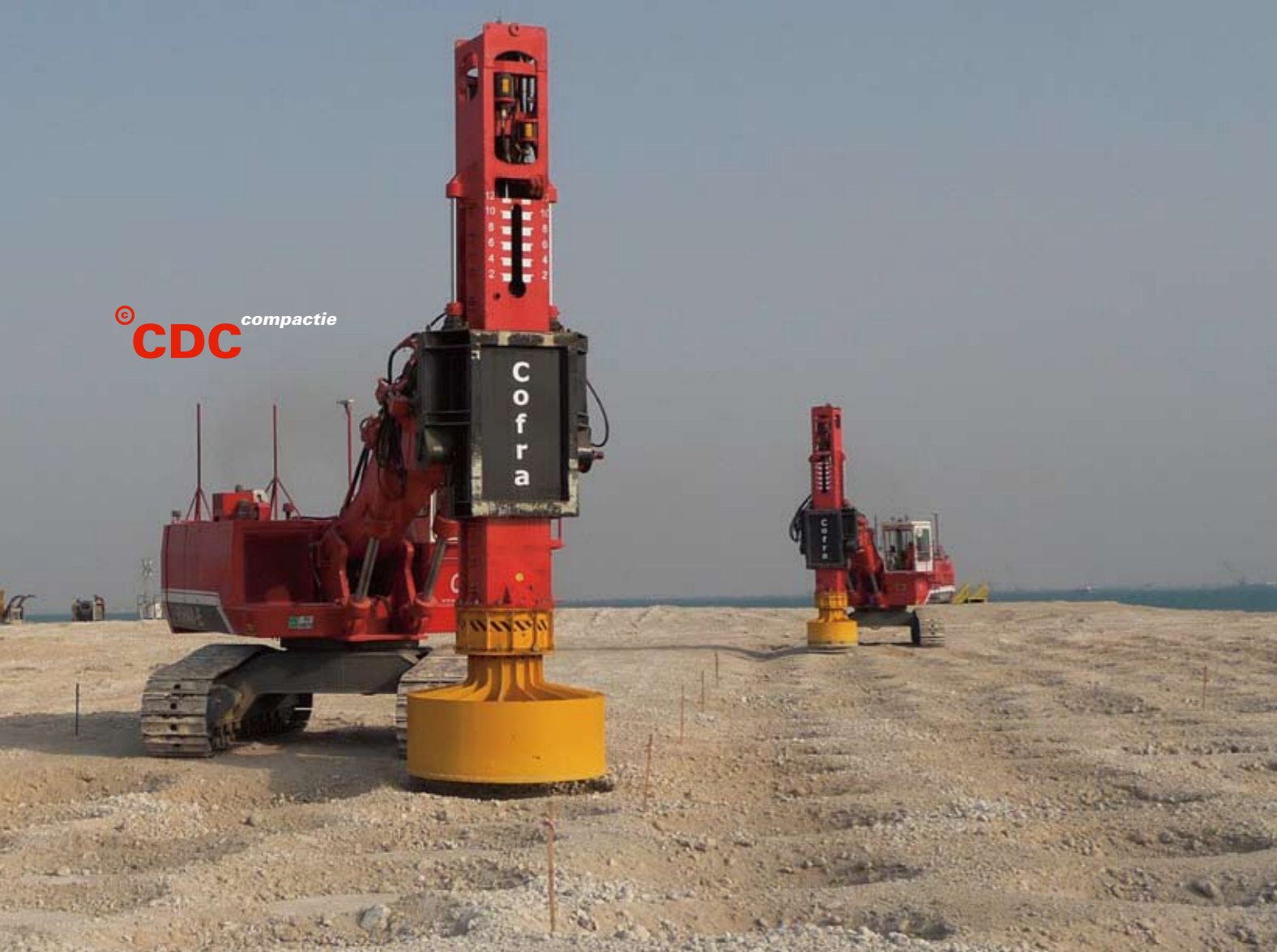
Compaction in a regular pattern
