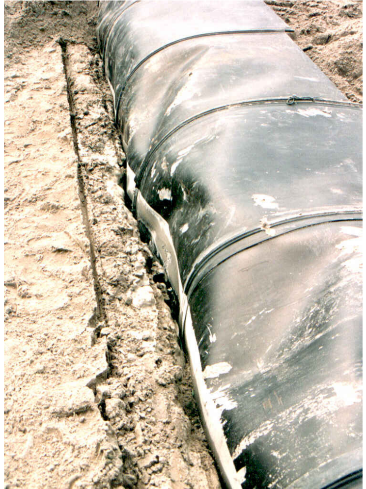
Figure 5 Installed Geolock panels
