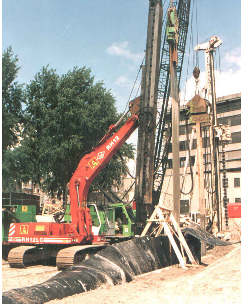
Figure 4 Drilling, bentonite trenching and Geolock installation rig on a row Rig
