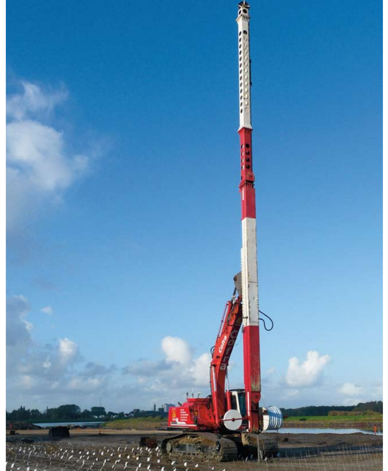
Installation of vertical drainage in the Weststrandweg project, Halfweg, The Netherlands
